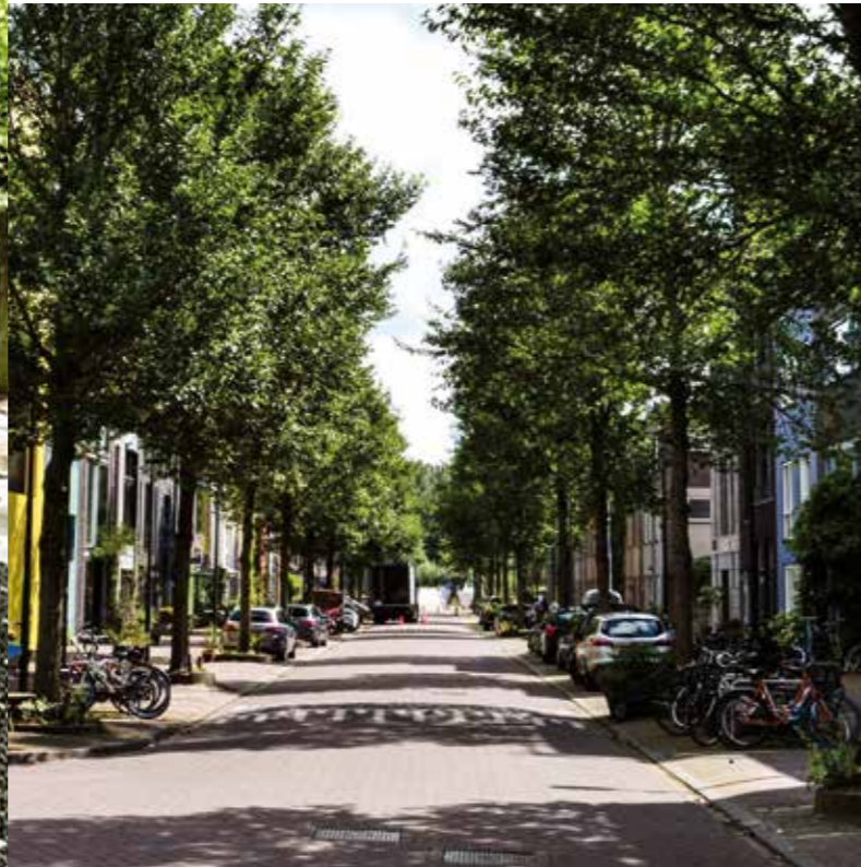
> Jan Olphert Vaillantlaan, Amsterdam, trees in a fully paved cityscape, 13 years after being planted in the Permavoid Sandwich Construction. Fantastic tree growth and zero pavement damage.
