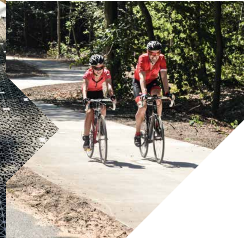
< Bicycle path Oosterhout where water detention and infiltration are of particular importance.
