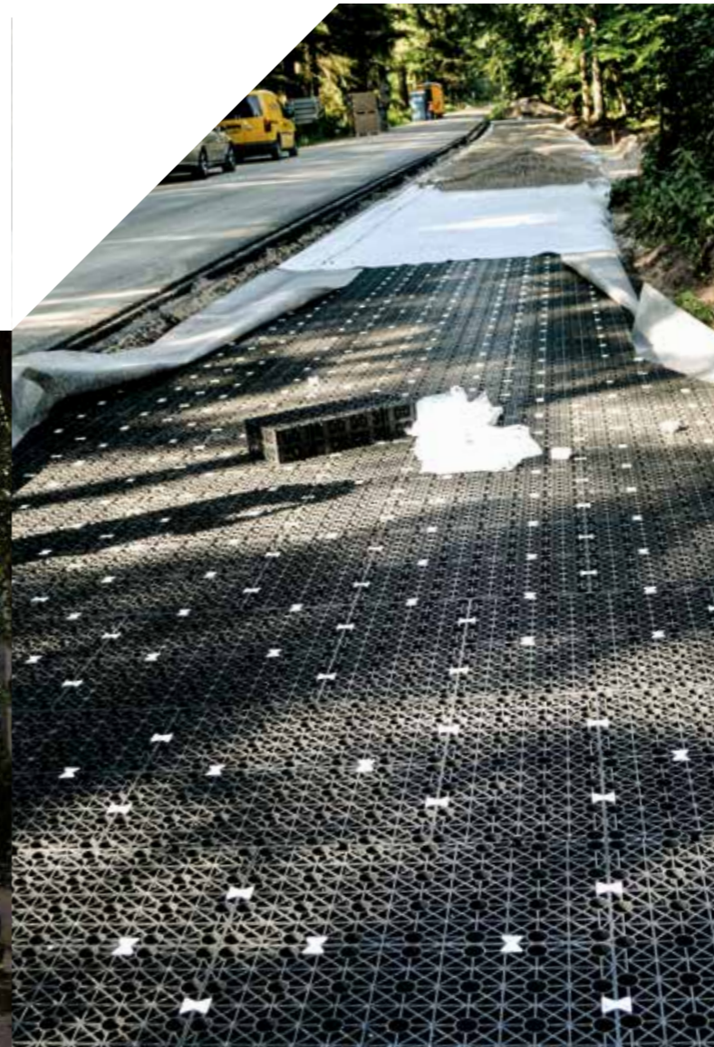
> Epe Heerdeweg. A floating bicycle path. For bicycle paths through existing green infrastructure, the shallow application and the lightweight construction are of particular importance in order to prevent damage to the rooted profile.
